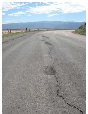
Figure 6. Hairline cracks along Parowan Gap road. Road patches indicate collapse of subsurface erosional pipes below the surface. View is to the east.
