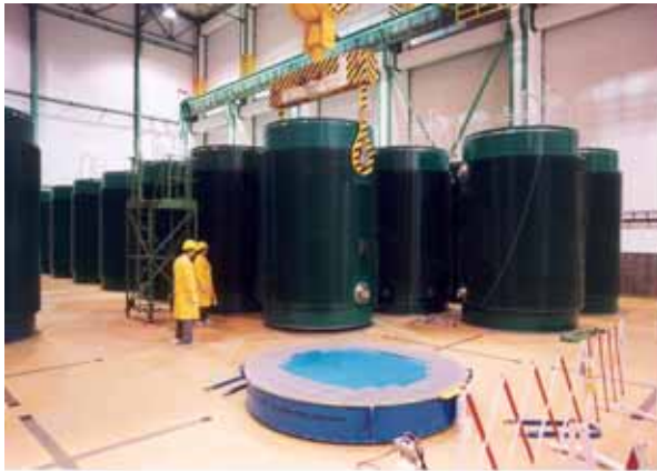
Dry Cask Storage
